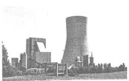
2. Many power plants cool their reactions with convective air flow through a hyperboliod tower. The shape increases air flow while minimizing construction
